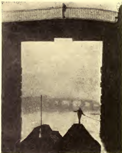
PASSING UNDER OLD BATTERSEA BRIDGE
